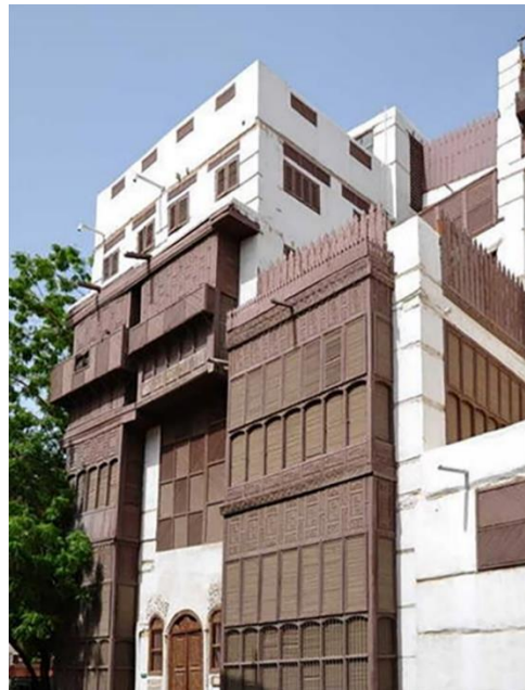
Fig. 5. Roshan in Old Jeddah.
