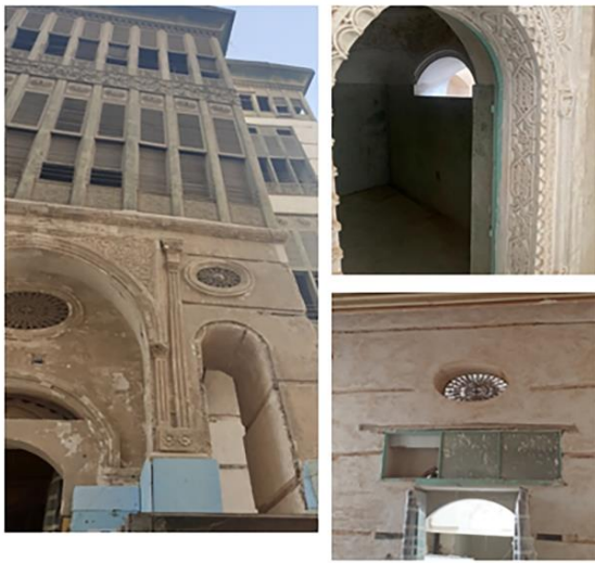
Fig. 10. Light pattern (Qamaria) Jokhdar House before restoration
